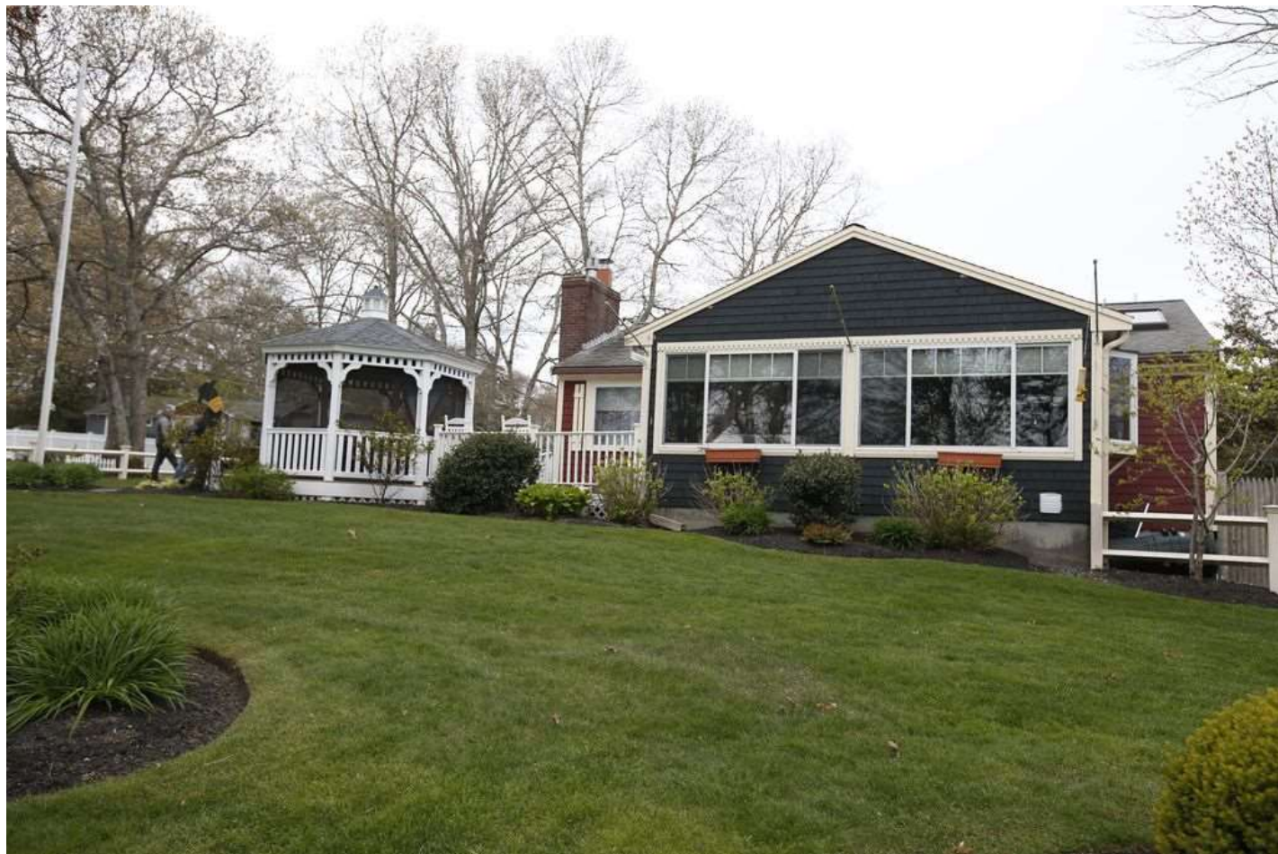
One of the homes that has had one of the new septic systems installed. JONATHAN WIGGS/GLOBE STAFF
