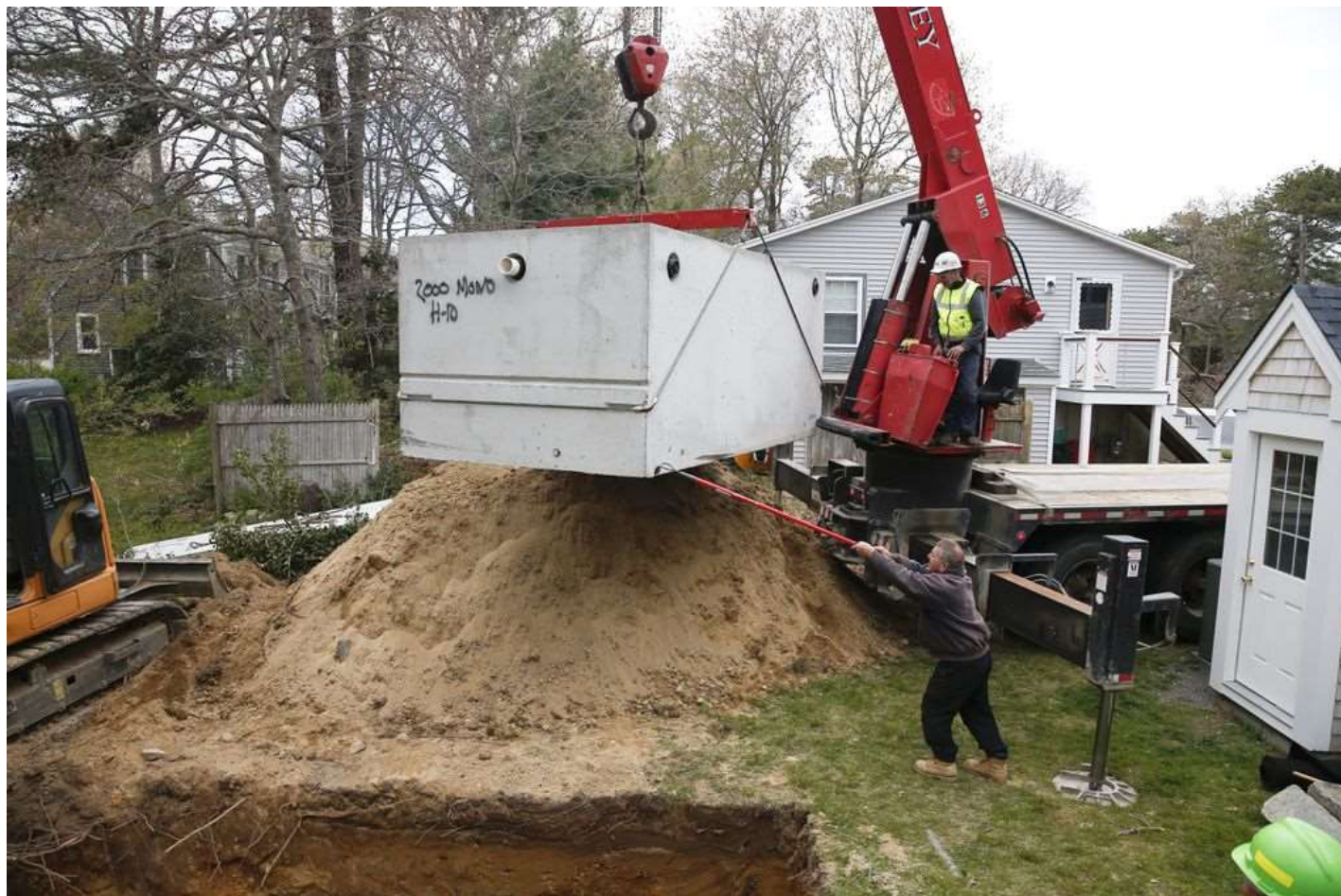
One of the new septic tanks was lowered into the ground. JONATHAN WIGGS/GLOBE STAFF
