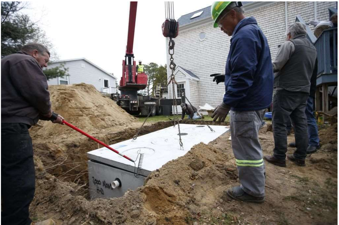
On Cape Cod, the Barnstable Clean Water Coalition installed a KleanTu septic systems in the Sandy Shores neighborhood around Shubael Pond.. JONATHAN WIGGS/GLOBE STAFF
