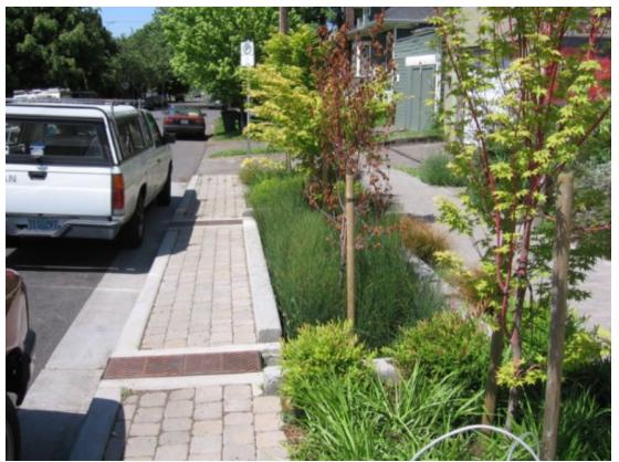
Bioretention cells provide stormwater treatment and offer environmental beautification to urban areas.
