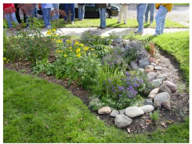
Bioretention cell in Massachusetts. Although small, this basin captures runoff from residential areas and helps protect water resources.
