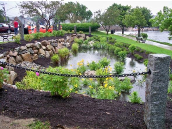
Beautiful bioretention basin at Water Street in Plymouth Center, Massachusetts, transforming stormwater from a potential source of pollution into a source of sustenance for plants and wildlife.
