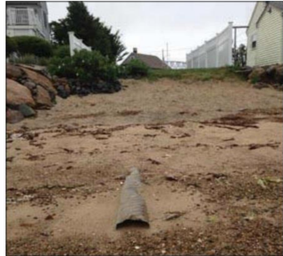
Figure 3. This stormwater outfall pipe no longer discharges to Fisherman's Cove after construction of stormwater BMPs.
